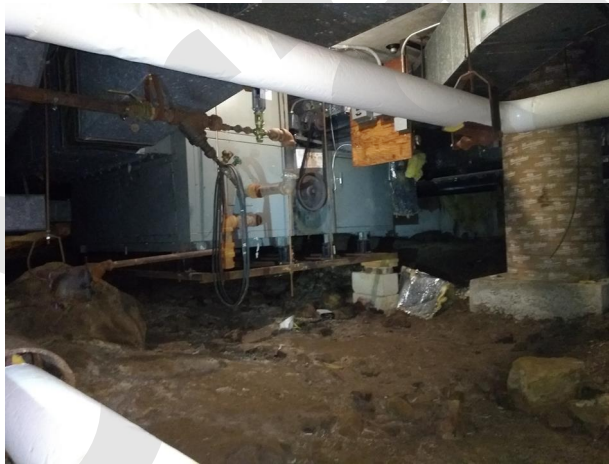
29. This Air Handling Unit in the crawl space is obsolete.
