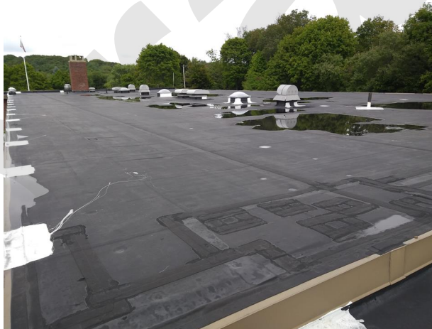
11. Rubber membrane roof has many areas of standing water and is extensively patched.
