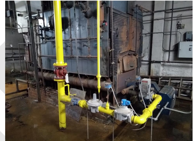
27. This 1975 era boiler is no longer being used.
