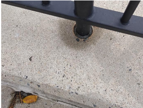
2. Rail posts do not have sealants and some sealants are failing.
